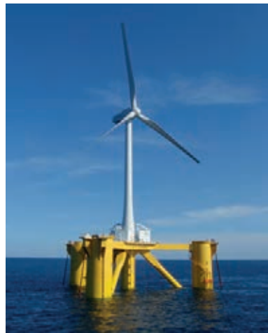
The 2MW experimental wind turbine that was floated off of Japan's northeast coast in 2013
