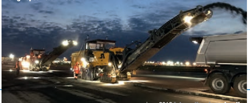
Milling machines working together using Topcon's 3D model
